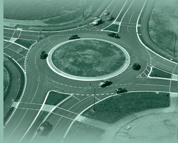
Over 5,000 roundabouts have been installed in Florida. Because of their safety and traffic calming features, roundabouts will continue to be an effective treatment and used in lieu of traffic signals or multi-way stop signs. Roundabout design features accommodate slower speeds while accommodating large vehicles like fire trucks and buses.
